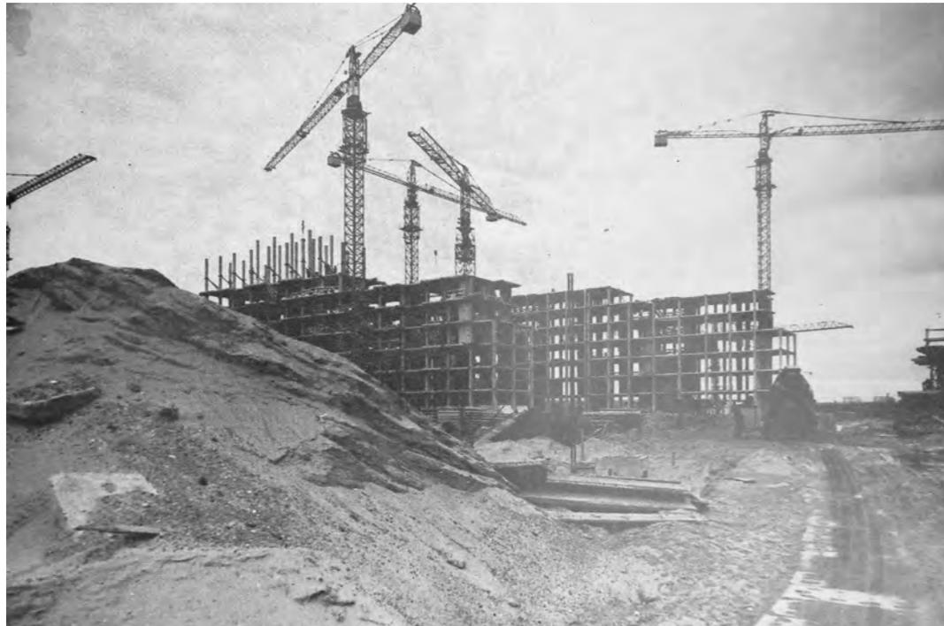
Construction phase of residential blocks 61-64 in New Belgrade using the 'IMS-Zeželj' industrialised building system
