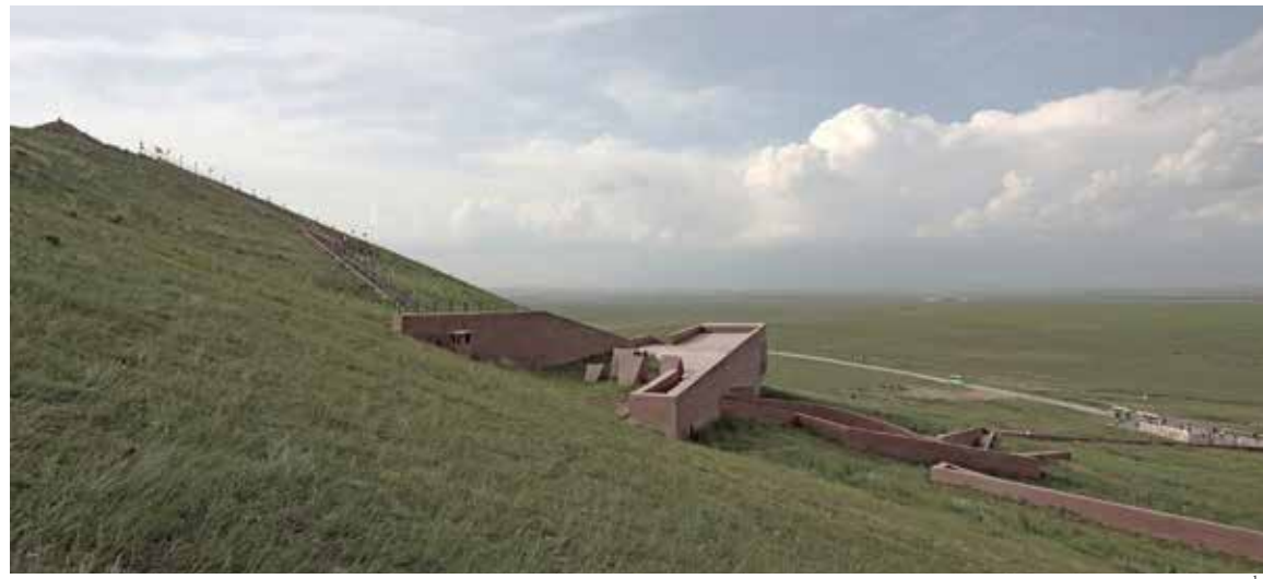
1. Semi aerial view from southwest 2-3. Distant View of Wulantai and Museum from Northwest Side 4. Distant View from East Side 5-6. Sunken courtyard 7. The axonometric drawing
