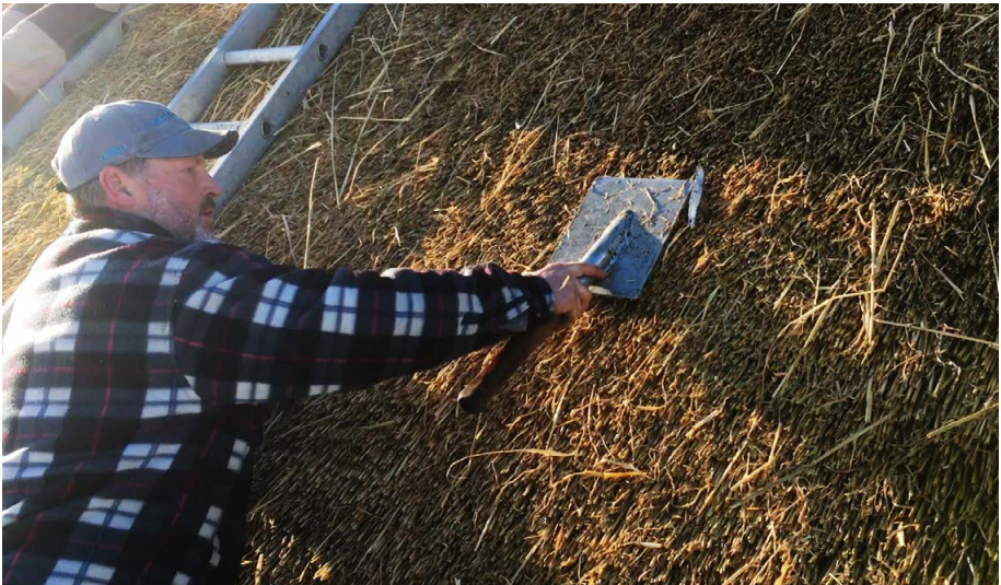
Thatcher using a Leggett, Scroggy Road, Glenavy © C60 Architects
