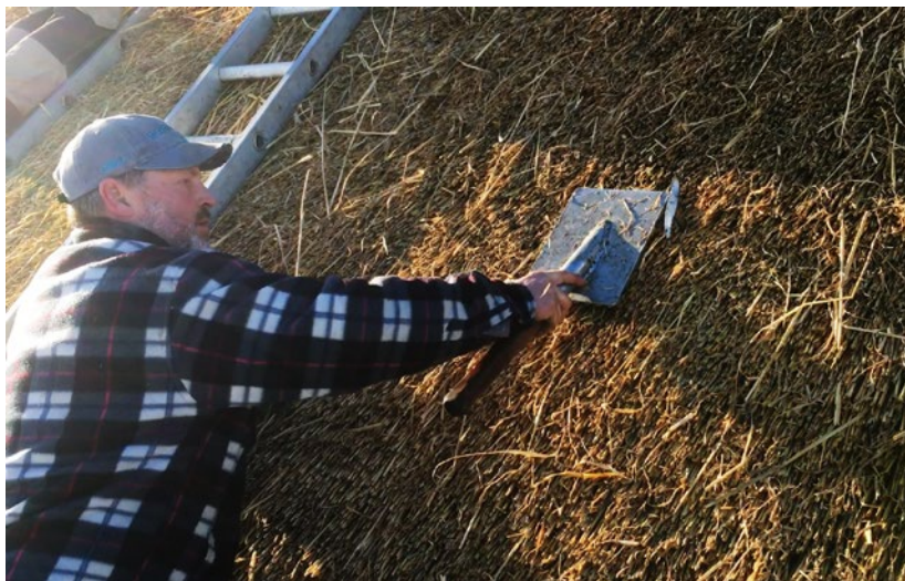
Thatcher using a Leggett, Scroggy Road, Glenavy © C60 Architects
