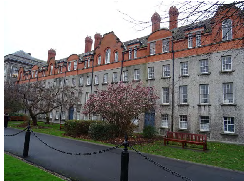
A contemporary view of the eastern elevation which shows how the building has changed over the years. The third floor was added in 1894-7 along with the present gabled arrangement. A coat of cement-based pebbledash was added to the elevation's Calp stone in the mid-20th century. © Carrig Conservation
