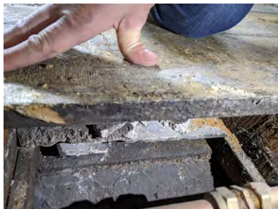
Historic slate covered with a lime and horsehair mix held in place by batten below the suspended timber floor. © Carrig Conservation
