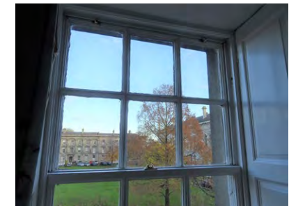
Early 18th-century sash window to the east elevation with thick glazing bars. © Carrig Conservation
