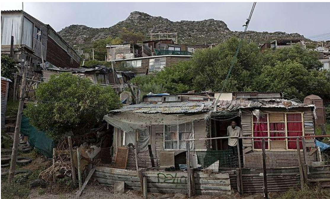
Fig 1: Hangberg before upgrading
