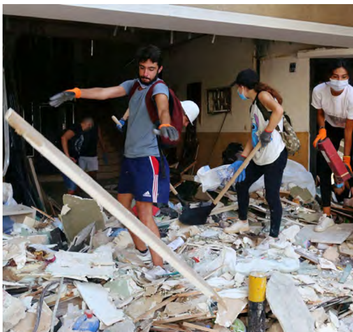
Volunteers clean rubble from the streets following blast. Credit: Aziz Taher
