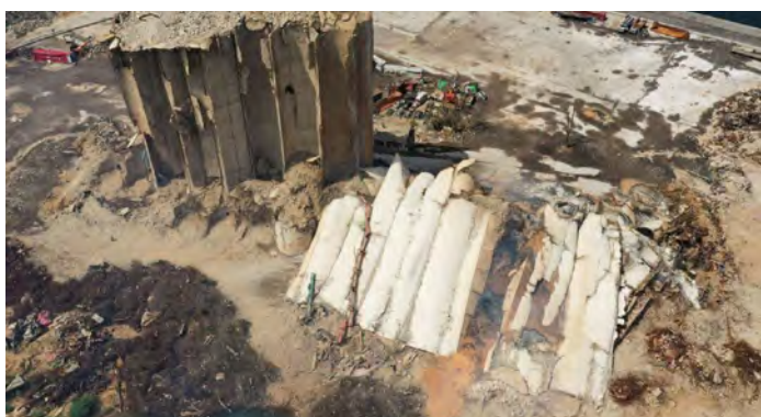
Collapsed northern section of the Beirut grain silos Credits: Issam Abdallah
