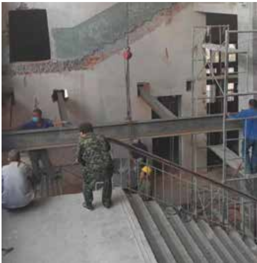
Construction of the mezzanine
