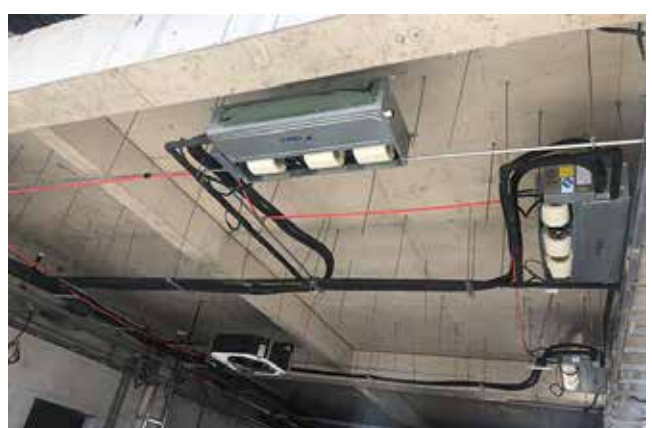
Air conditioning units installed on the ceiling to blow downwards
