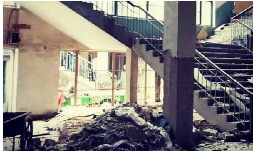
Exposing the concrete columns
