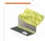
Masonry Wall Below Planted Slope
