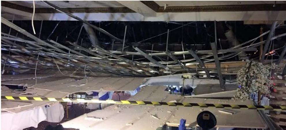
Figure 3. Inadequate fixings. Picture credit: West Midlands Ambulance Service
