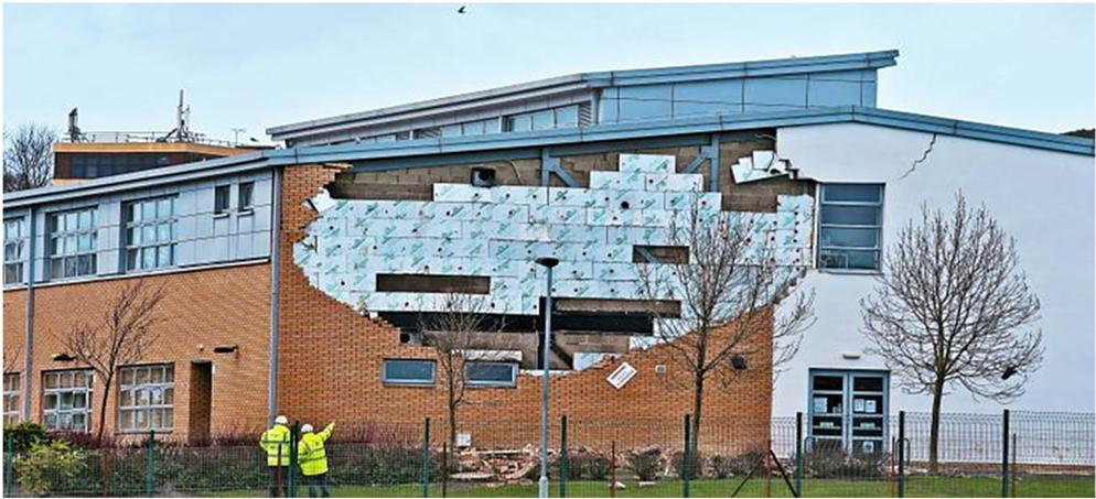
Figure 1. Incorrectly fixed cavity wall ties and omission of lateral restraint fixings.
