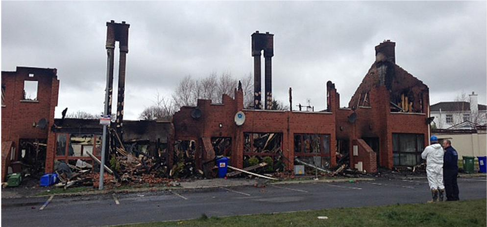
Figure 2. Fire stopping / compartmentation omitted.
