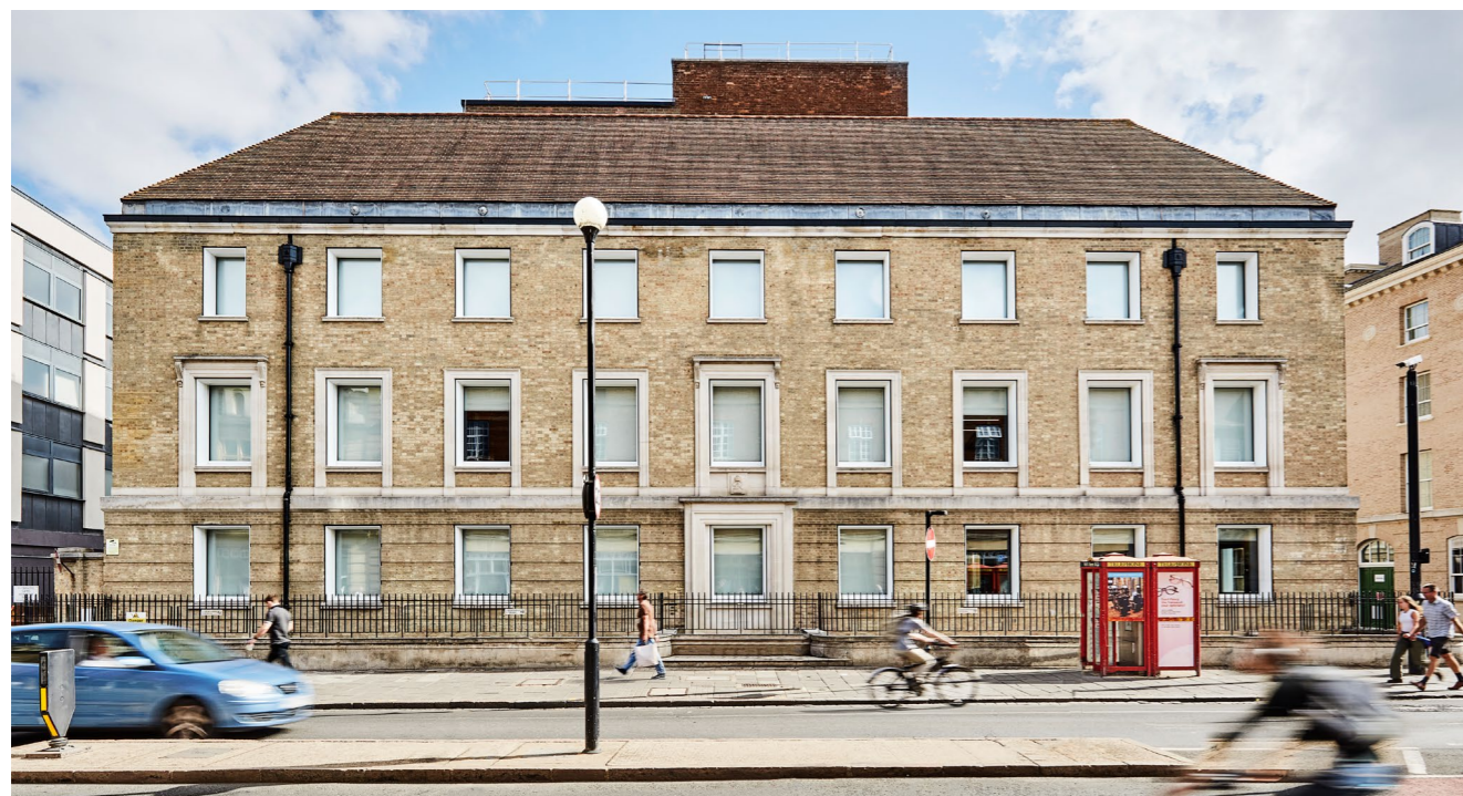
Entopia Building, Deep Retrofit Office, Certified EnerPHit Archetype Image © SOLK Photography Ltd
