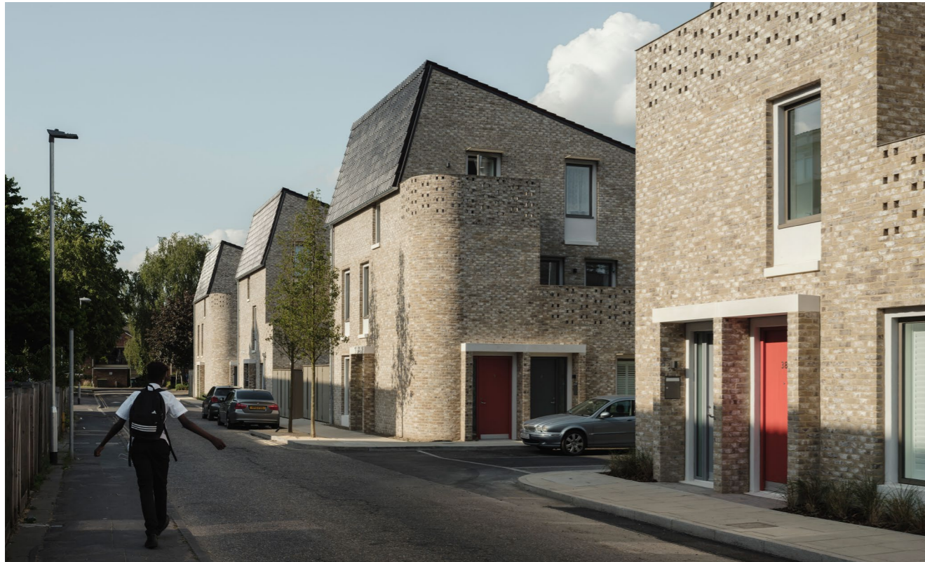
Goldsmith Street, Social Housing, Certified Passivhaus Mikhail Richman Image © Tim Crocker
