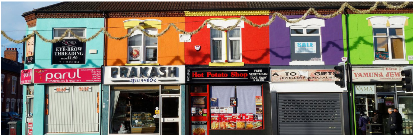
Brightly painted buildings on 'the Golden Mile' in Leicester. Photo: ANDRYPHOT | Alamy Stock Photo
