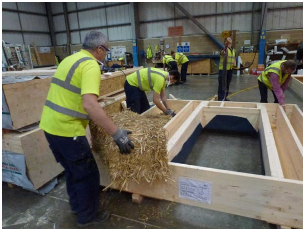
Building a ModCell wall panel © ModCell
