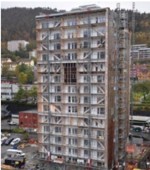
14 storey Treet building in Bergen, Norway © Rob Foster
