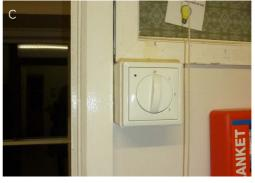
Figure 20 (A) First floor windows - fully openable giving good access to original sash windows (B) Ceremony room windows - windows opening hindered by furniture (C) Electric window switches - the electric windows they control are not visible from the switch location hence no indication of system response
