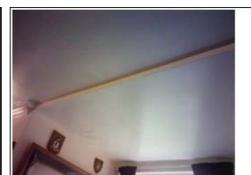
Figure 5 Ground floor room showing thermal anomalies on the ceiling which is potentially due to poor insulation of the pitched roof above the windows
