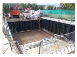
Figure 3.12 Construction of the can-float base
