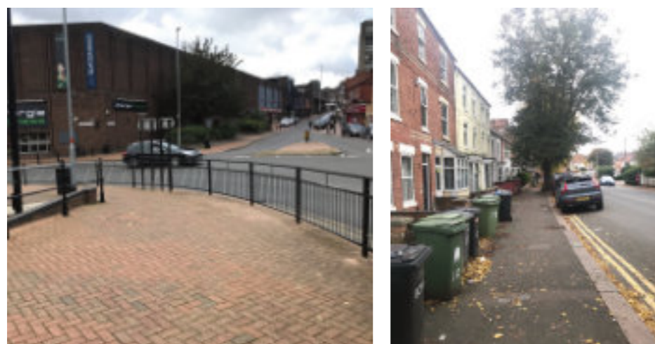
Brick paved surface extends only as far as the Town Gateway, then becomes asphalt; bins are a problem if sufficient storage is not provided
