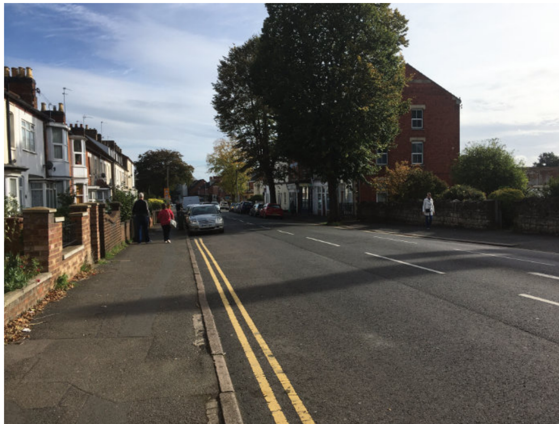
Surfacing of both carriageway and footpaths in black asphalt tends to emphasise street as vehicle corridor over street as place.
