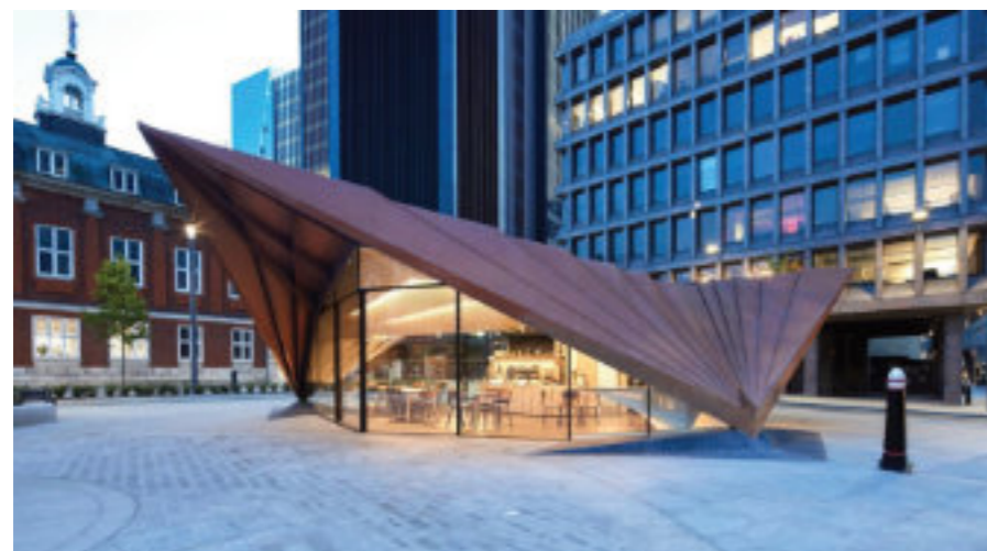
Portsoken Pavilion, City of London [Make Architects]
