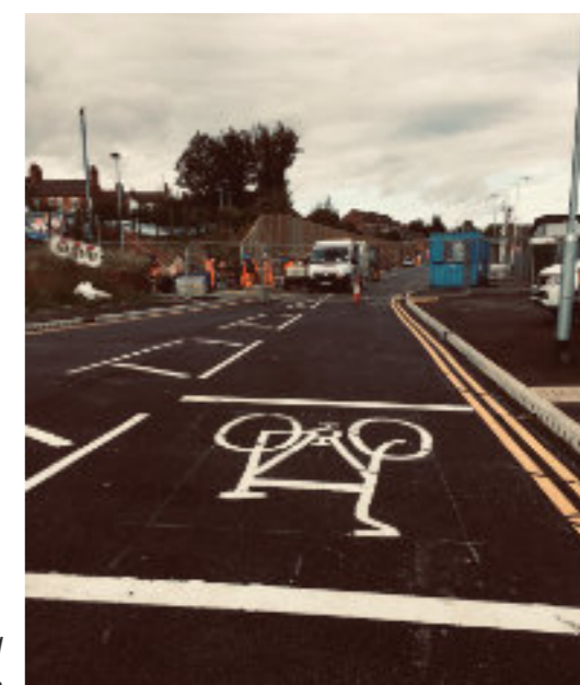
Right - view north along Route 4, nearing completion
