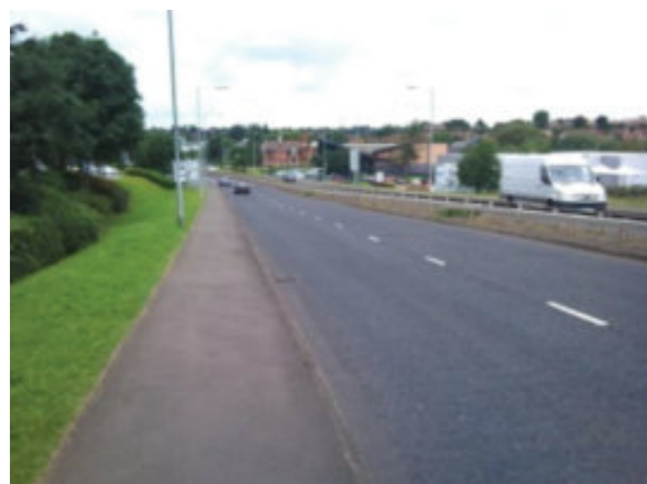
USS example of a radial route hostile to non- vehicular users [Kettering]
