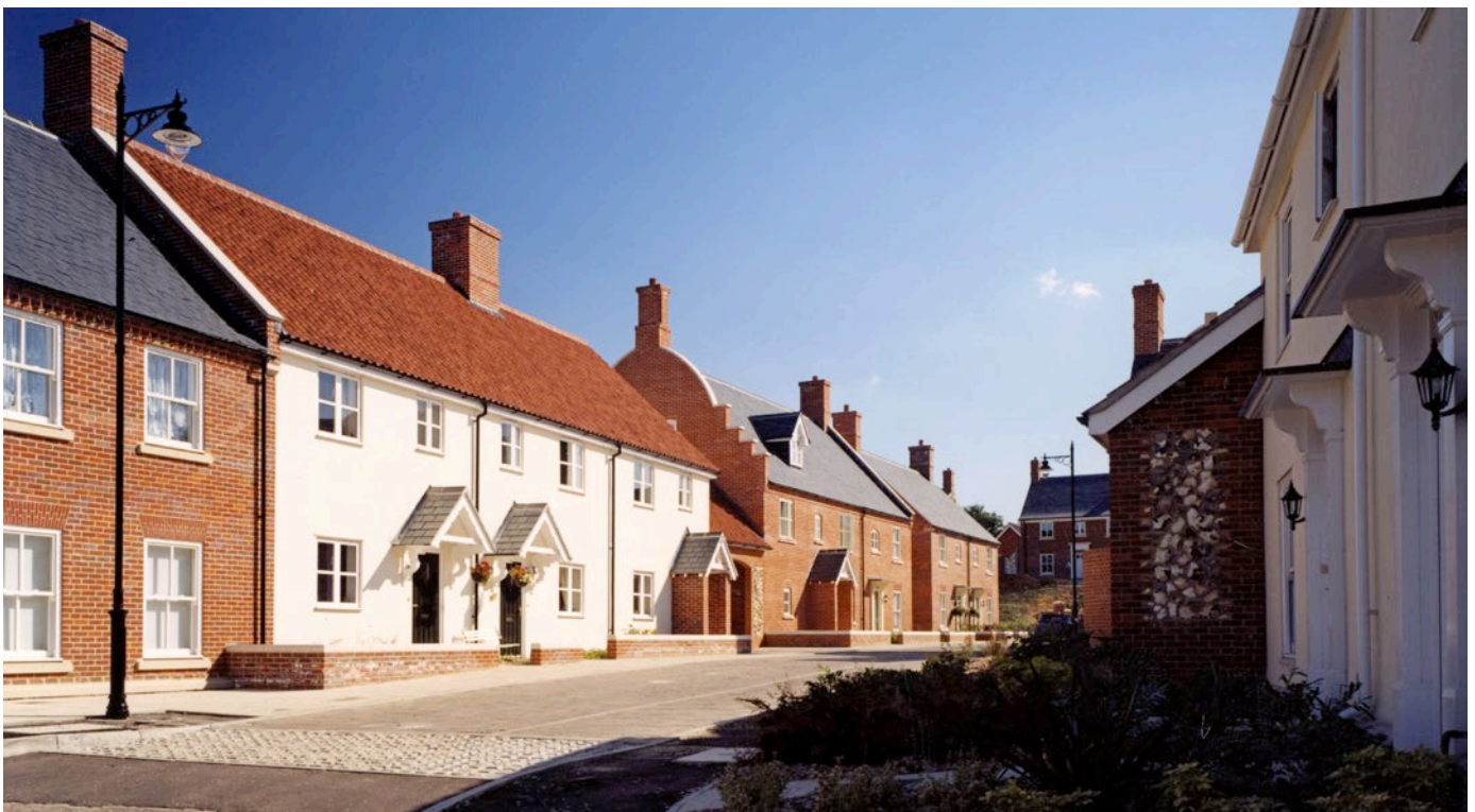
Trowse Newton The focus of the scheme is a crescent of houses at the end of the village street, incorporating the existing public house.
