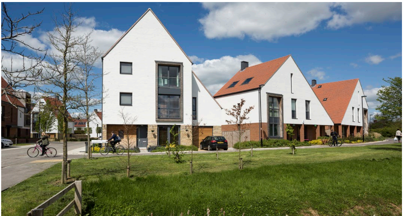
Derwenthorpe A network of pedestrian and cycle routes cross the site allowing easy access between neighbourhoods and into the centre of York.
