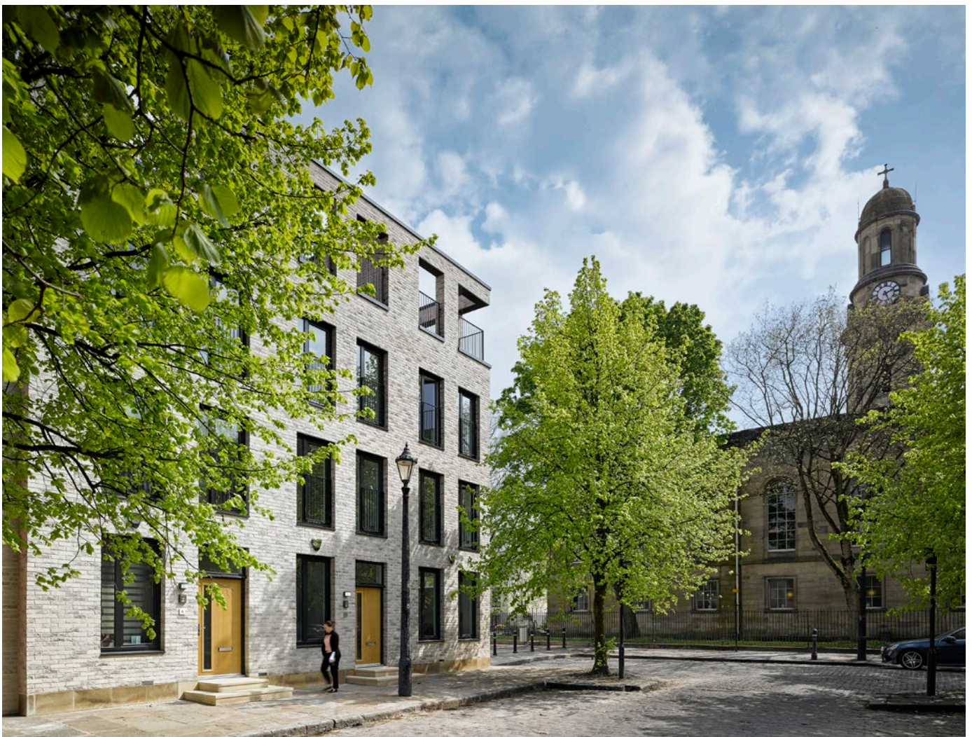
Timekeepers Square "The landscaping is well designed and executed, with fine natural materials and good detailing."
