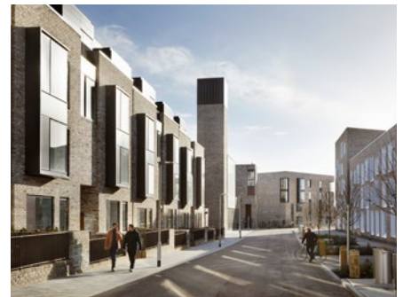
Eddington A central energy centre is a distinctive element which references the tradition of Cambridge chimneys, giving a strong identity to the scheme.
