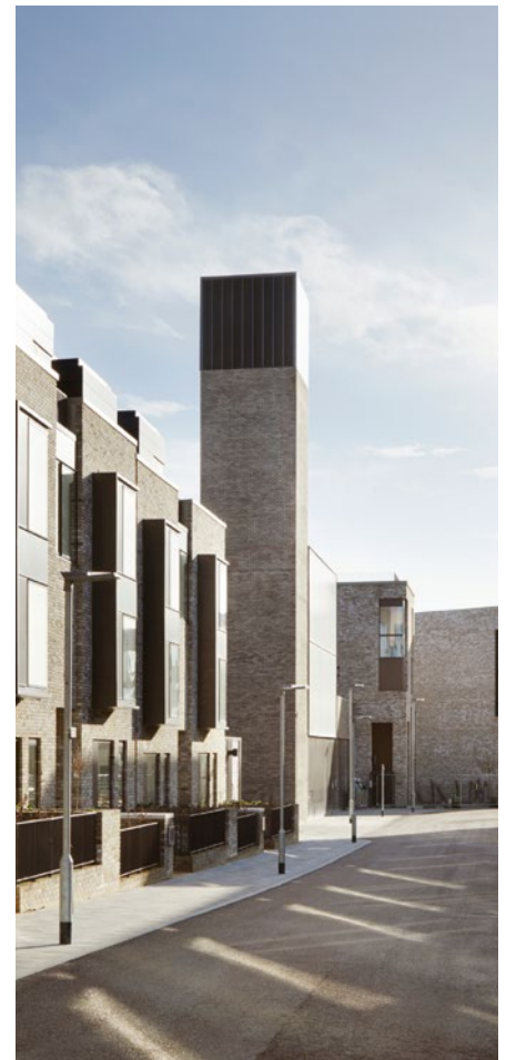
Eddington A central Combined Heat and Power energy centre serves the entire development.
