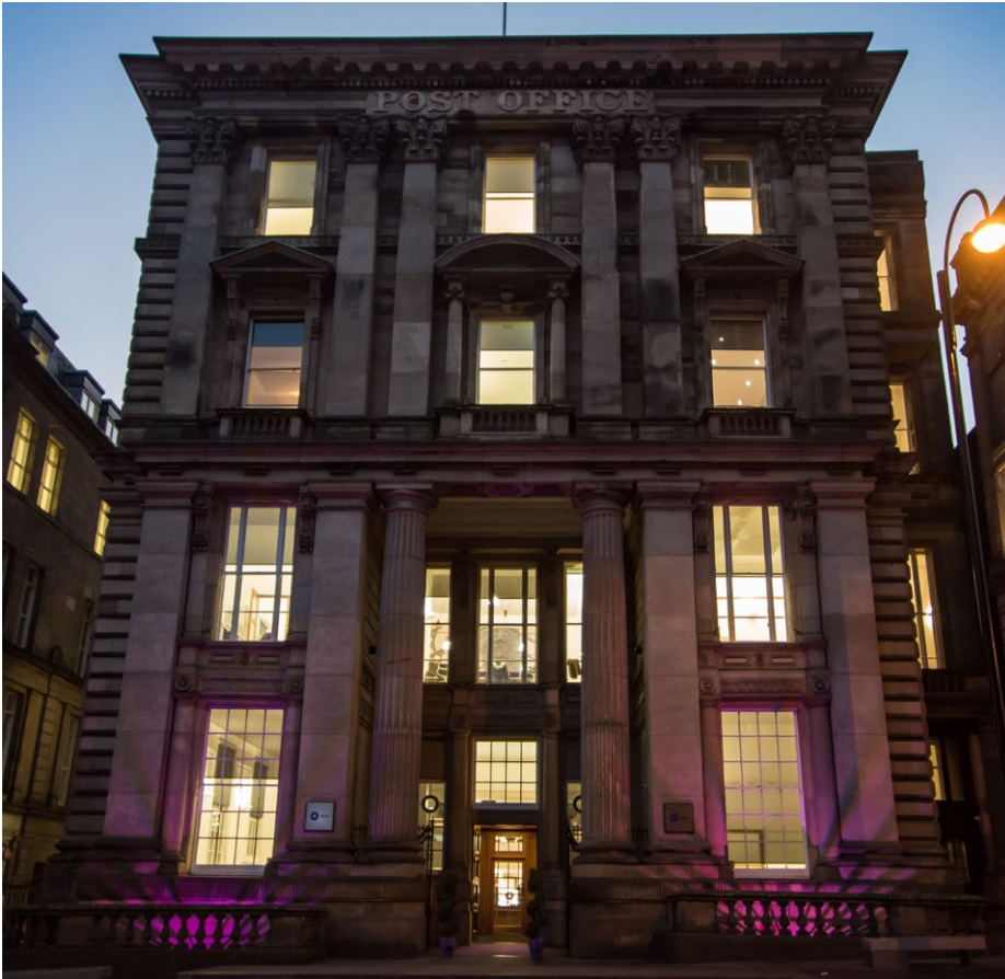
The successful £5.8m redevelopment of the NBS head office at the Grade II listed Old Post Office building in Newcastle demonstrated the value of NBS BIM services and tools. Credit: The Bigger Picture Agency Ltd.
